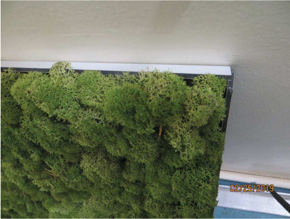
Figure 3 – Protrusion of organic material from tray
