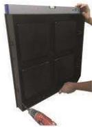
E. Going into Studs: Sometimes, the hole is located over a stud. Just use the electric drill and the correct size driver to drive a self-tapping metal screw into aluminum studs or a lag screw into wood studs. Use caution not to over tighten so as not to damage the frame.
